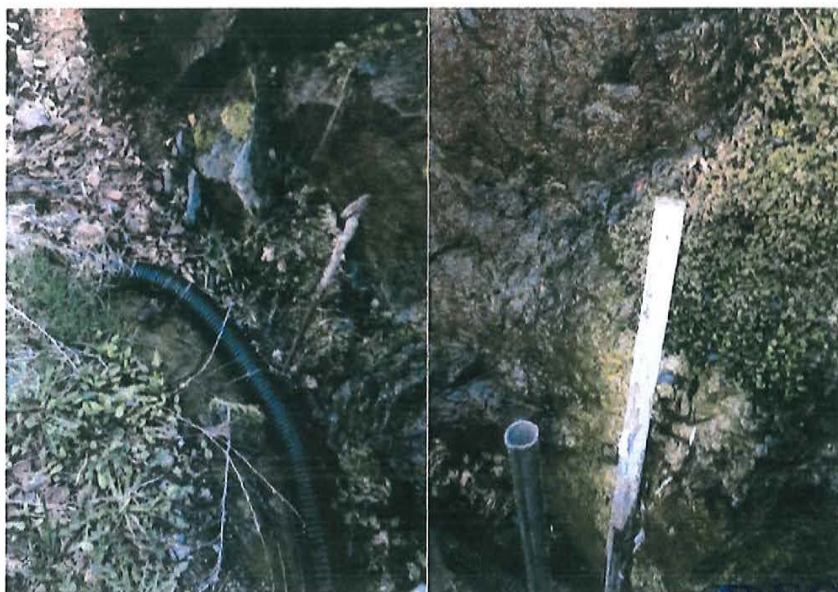
Photo 2: Diversion of the groundwater seepage to the south, off the site, facing west, April 16, 2015.
